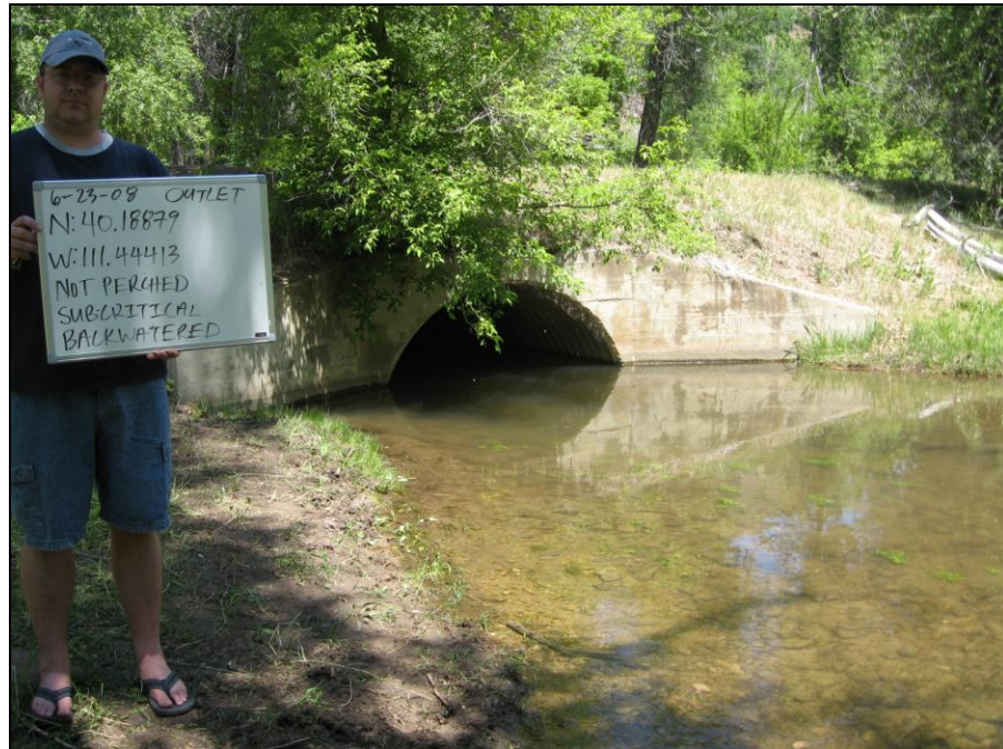
Figure 4-2: Hydraulic Evaluation Photo Taken at the Outlet
