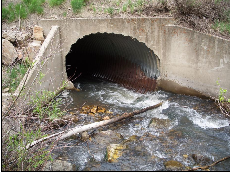
Figure 5-42: Hydraulic Jump Just Upstream of Inlet
