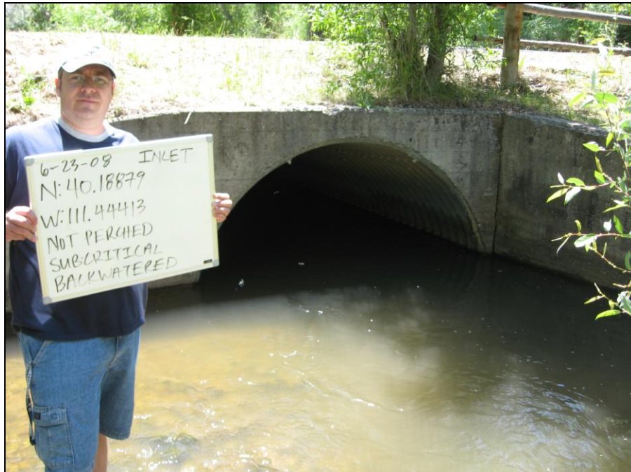
Figure 3-4: Hydraulic Evaluation Photo of a Culvert Inlet
