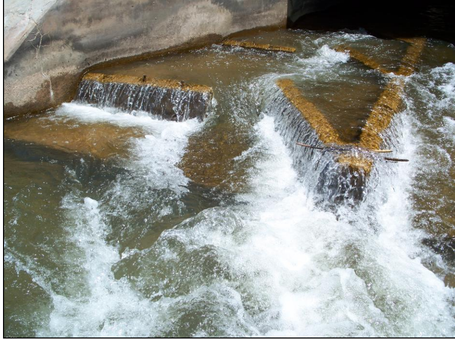
Figure 5-11: Photo at Outlet of Fish Baffles
