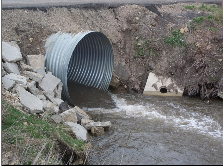
Figure 5-44: Hydraulic Jump Just Downstream of Outlet
