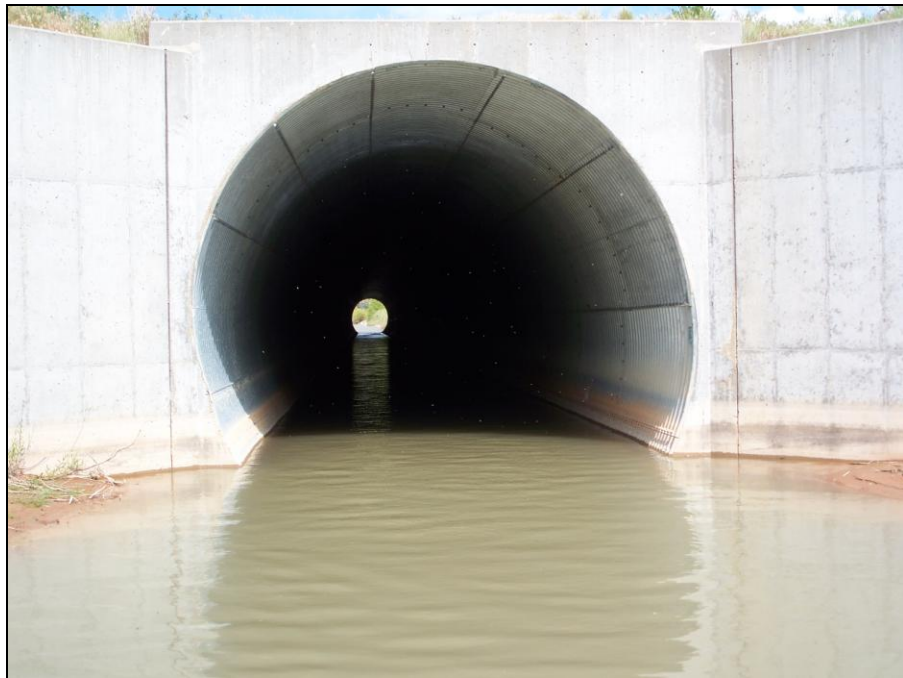
Figure 6-9: Soldier Creek Culvert Outlet (Soldier Creek Field Verification Site)
