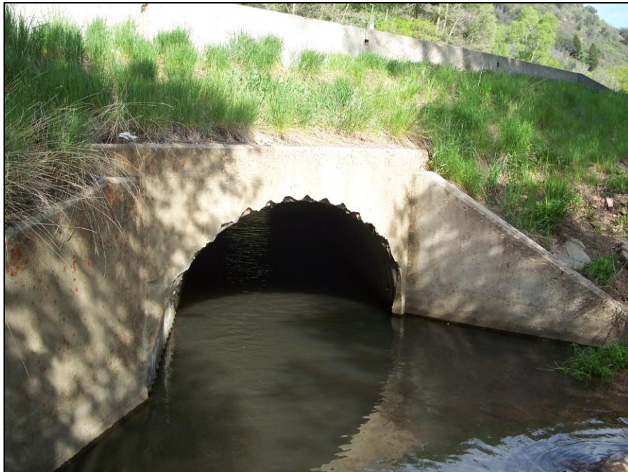
Figure 4-13: Outlet of Backwatered Culvert #3
