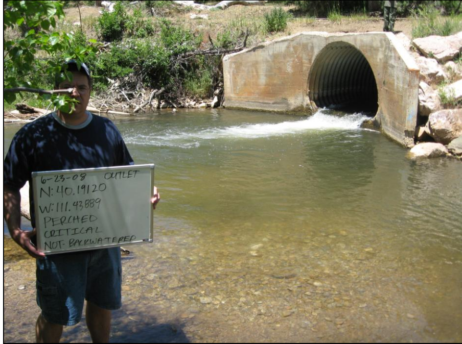
Figure 3-5: Hydraulic Evaluation Photo of a Culvert Outlet
