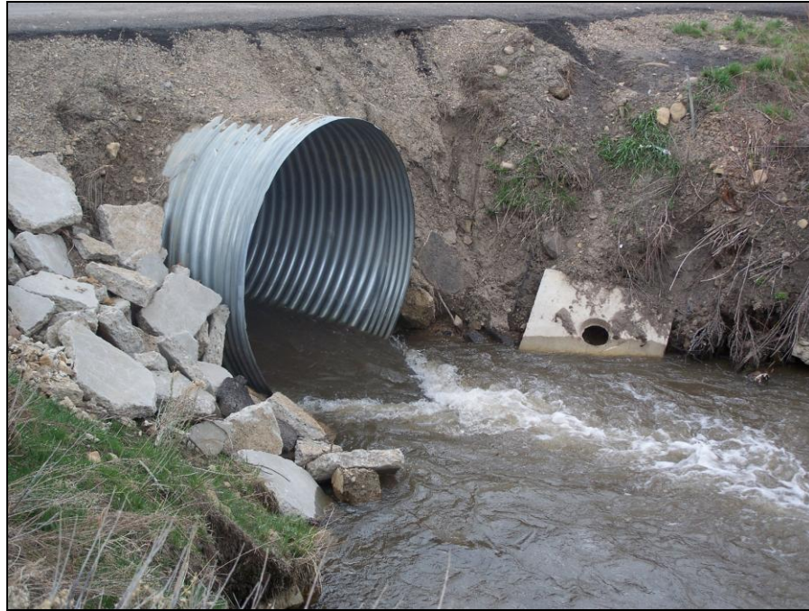
Figure 4-14: Elevated Outlet
