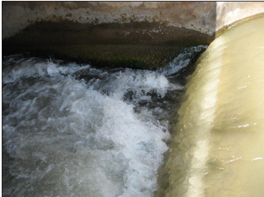
Figure 5-16: Detailed View of Spillway at Inlet
