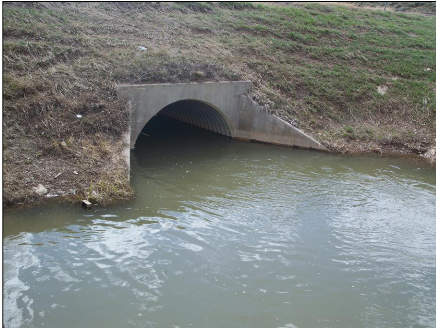
Figure 4-9: Outlet of Backwatered Culvert #1
