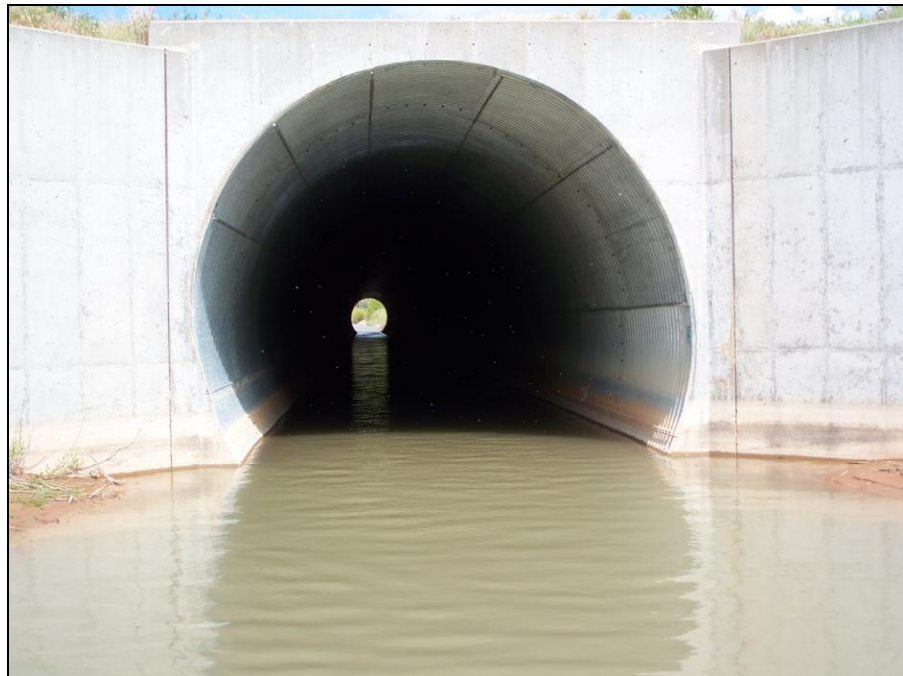
Figure 4-11: Outlet of Backwatered Culvert #2
