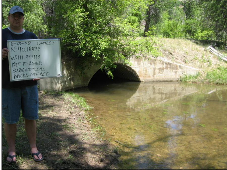
Figure 3-3: Hydraulic Evaluation Photo of a Culvert Outlet
