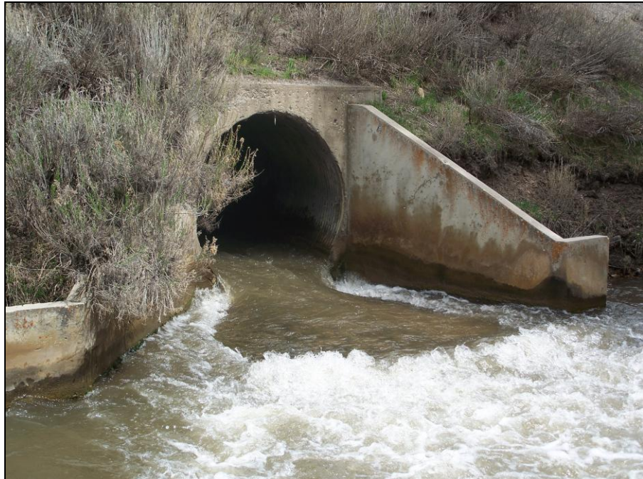
Figure 5-45: Hydraulic Jump at End of Outlet Apron
