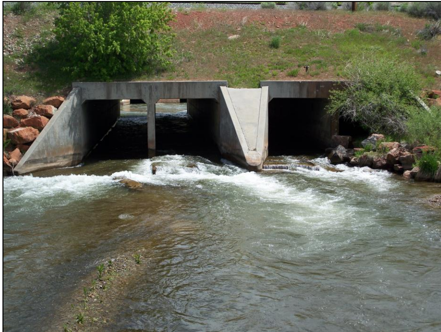
Figure 6-3: Diamond Fork Culvert #1 Outlet (Diamond Fork Field Verification Site)
