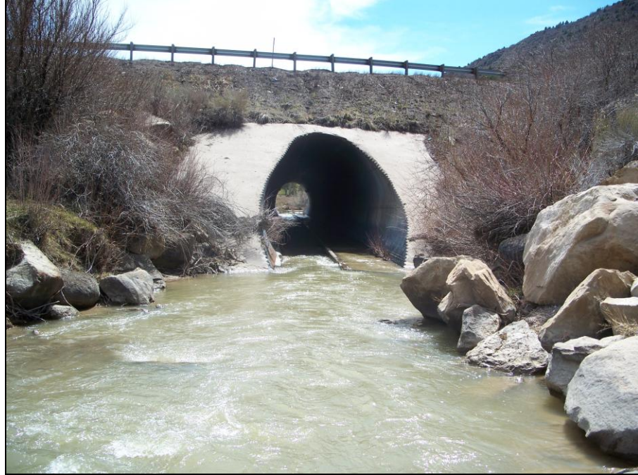
Figure 5-18: Photo of Inlet From 25 Feet
