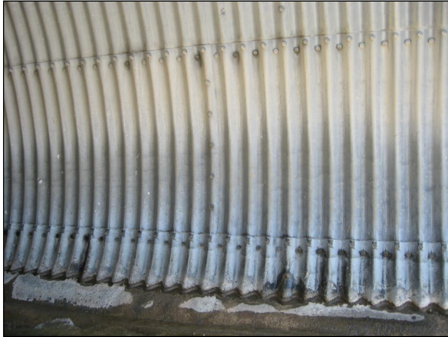
Figure 5-34: Plated Culvert
