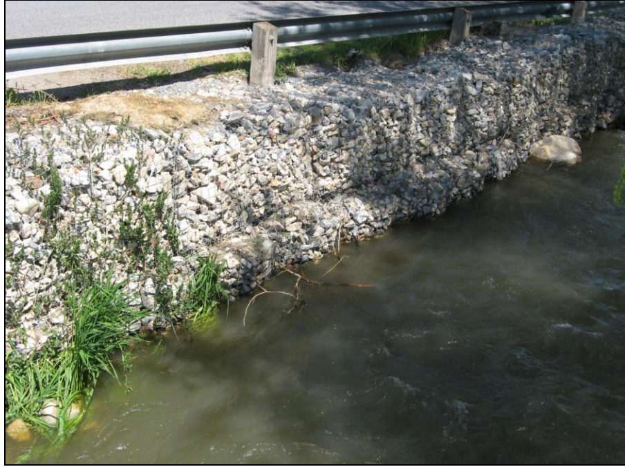
Figure 5-24: Gabion Wall
