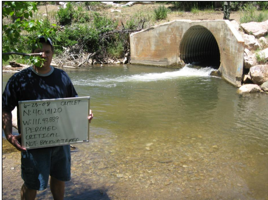
Figure 4-4: Hydraulic Evaluation Photo Taken at the Outlet
