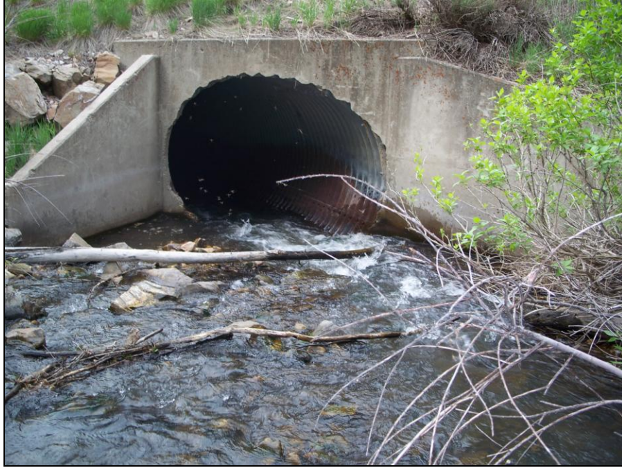
Figure 6-14: Daniel's Creek Culvert #2 Inlet (Daniels Creek Field Verification Site)
