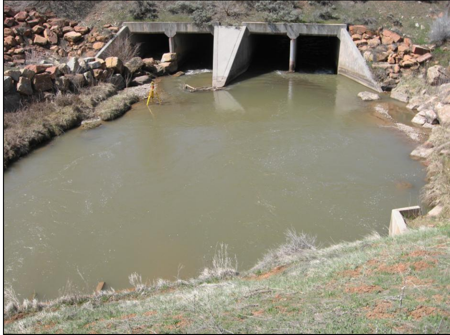
Figure 6-4: Diamond Fork Culvert #1 Inlet (Diamond Fork Field Verification Site)
