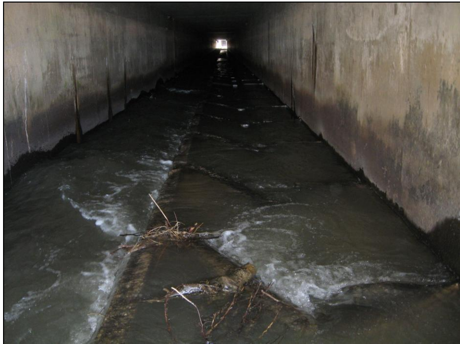
Figure 5-12: Photo of Fish Baffles Mid-Culvert
