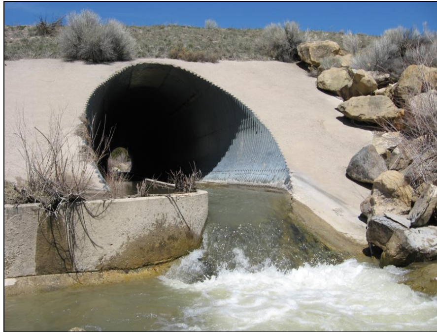
Figure 4-17: Elevated Outlet
