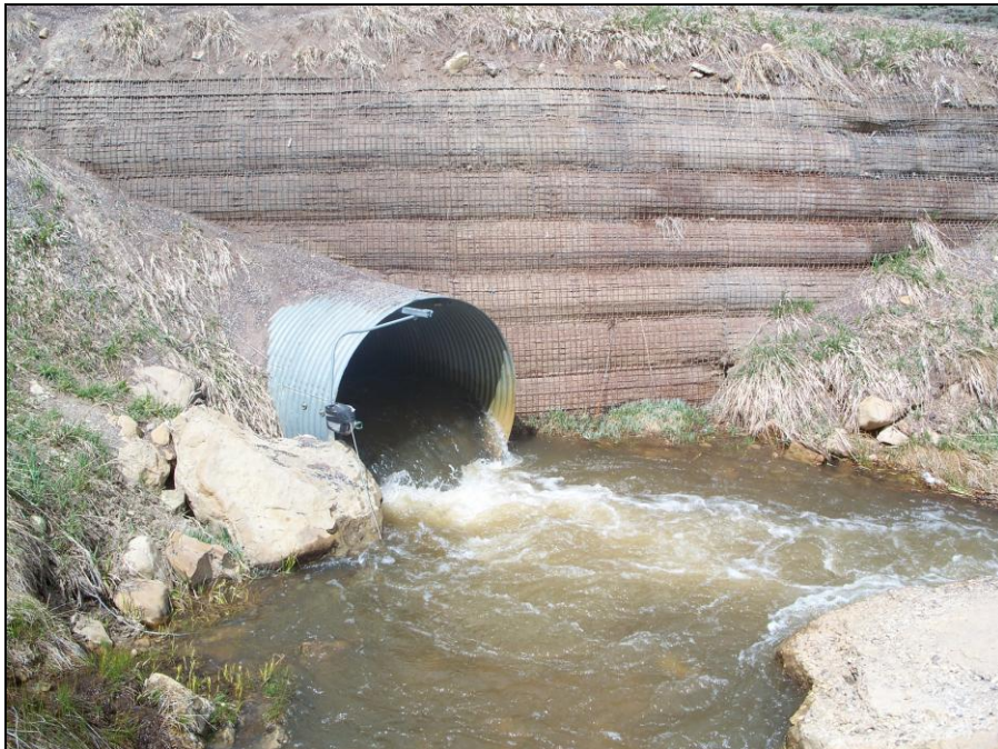
Figure 5-23: Gabion Wall
